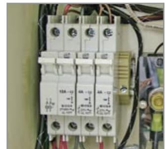
Figure 11.1.4 – Control Panel Breaker
