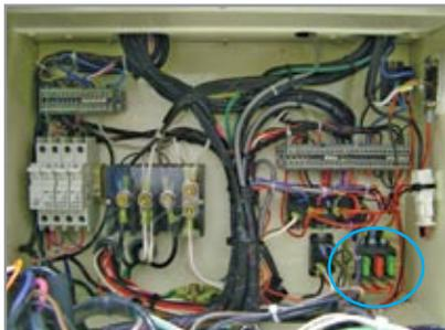
Figure 11.1.2 – Control Panel Fuse location
