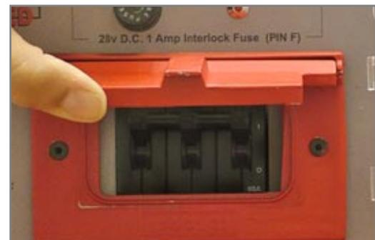
Figure 5.2.4 - 400Hz AC Input Circuit Breaker set to the “ON” position.
