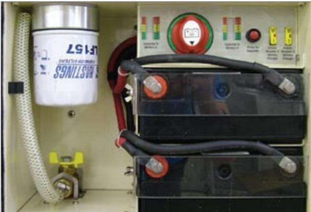
Figure 13: Oil Filter, 12 Volt Batteries, and Battery Selector Control Panel
