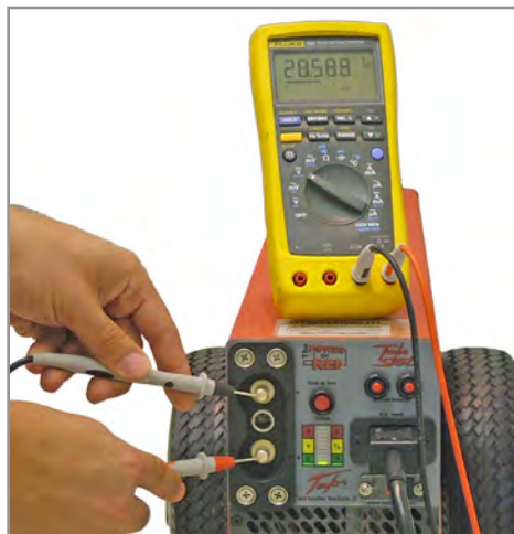
Figure 7.2.3 – Testing DC Receptacle
